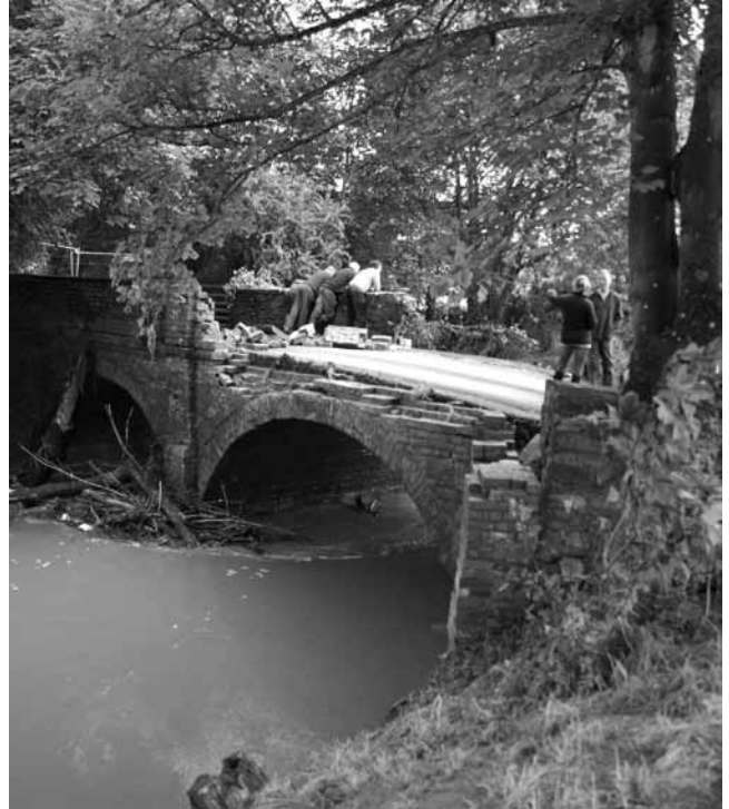
Upstream the damage seems greater, with the main structure showing evidence of battering.
