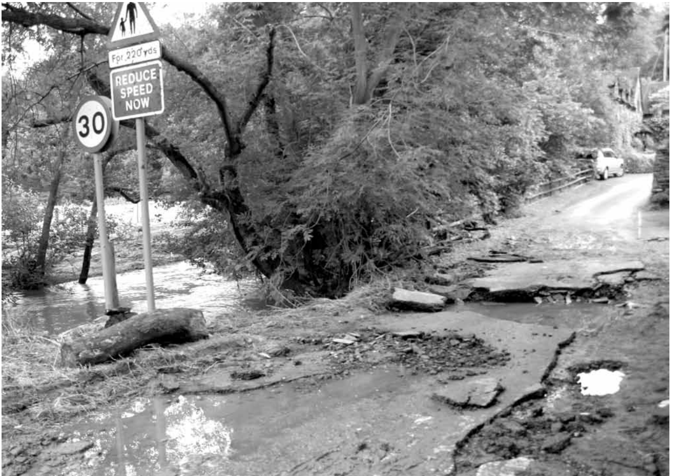
At the bottom of Ronhill the road surface has been torn up by the pressure of water draining down off the neighbouring hill and the traffic signs stand like isolated sentries on their bases, the bank around washed away by the flood. What is normally just a trickling stream turned into a torrent and inflicted this level of damage after hours of heavy rain overwhelmed the drainage system.
