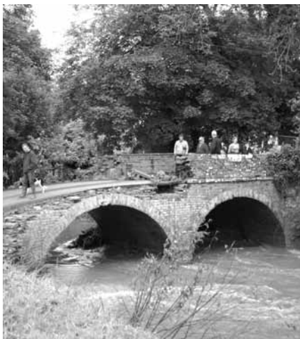
The Grade 2 listed bridge at Neen Sollars, one of the victims of the July 14th moonsoon. See Page 35
