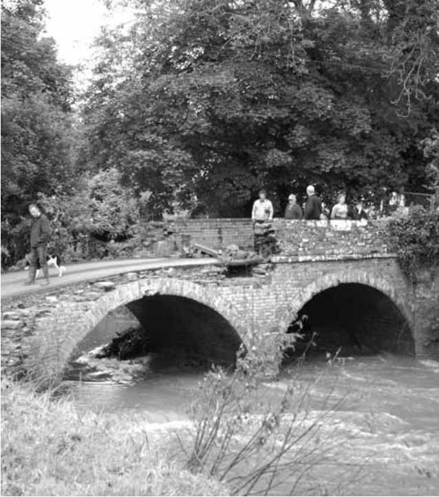
Downstream from the Neen Sollars bridge, with only foot traffic allowed as the damage is assessed.
